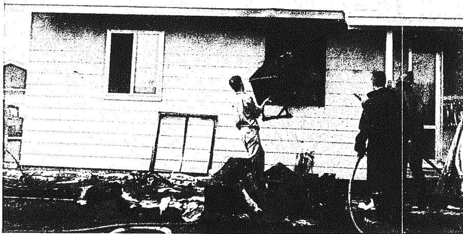
Pictured above is debris being removed from fire-damaged house
