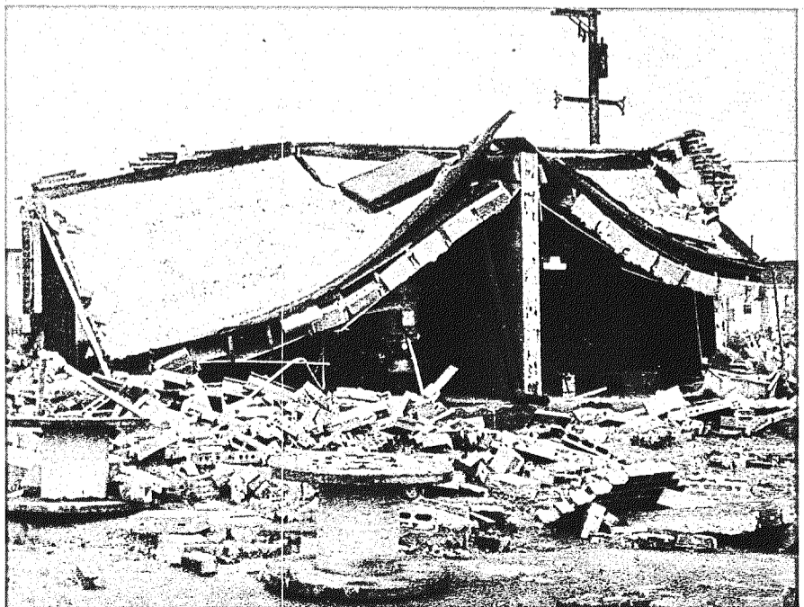
Pictured above is the Woodridge Sewer and Water Co. pump house after an explosion Aug. 6 caused an estimated $20,000 damage with a loss of 165,000 gal. of water.
